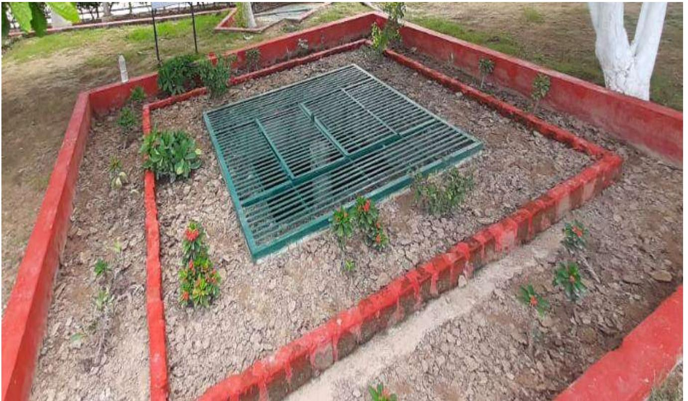
**An Example of Rain Water harvesting underground well which may be constructed in GSC, Naya Nangal Campus**
